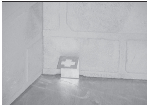
Figure 8.8 Grate Retaining Bracket in Place
